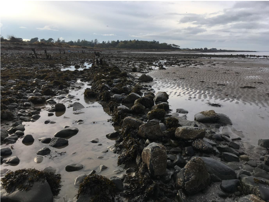
Plate 2: Target Note 1: Low stone wall and wooden pilings at southern corner of Landfall Option A.
